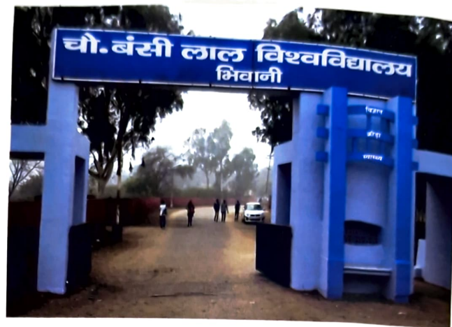
University Gate after Renovation
